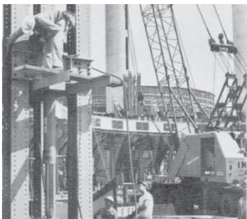
Interior Construction on New York State Progress Report #9, September 26, 1963
