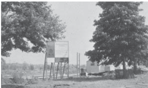
Construction on New York State Pavilion Progress Report #6, September 12, 1962
