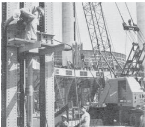
Interior Construction on New York State Progress Report #9, September 26, 1963
