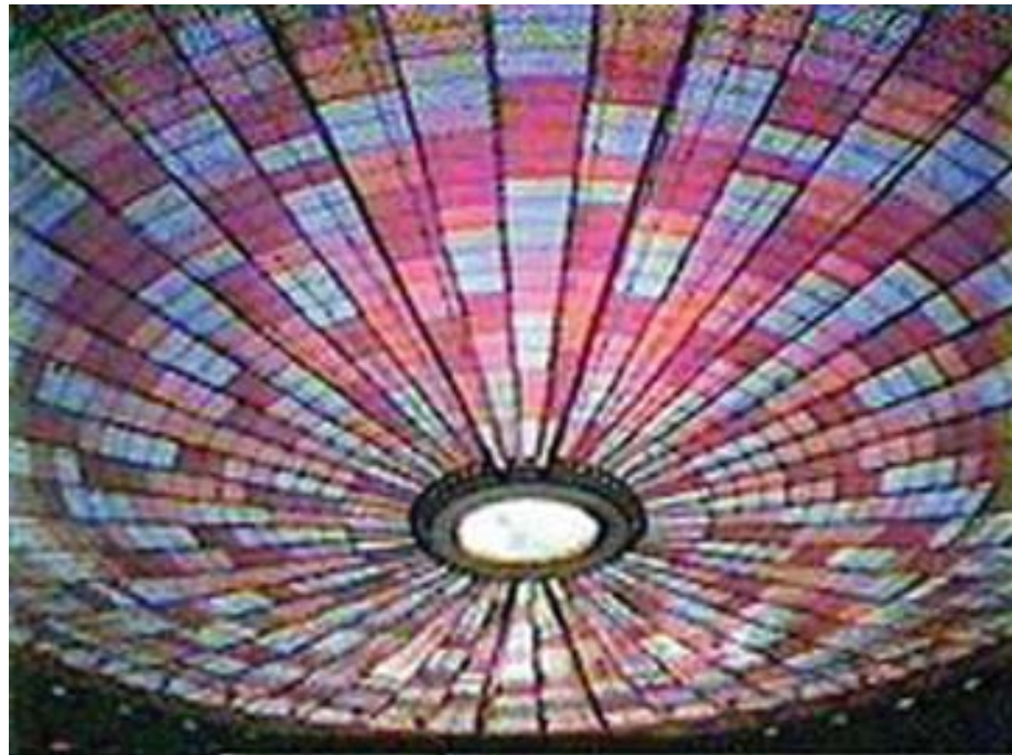
Interior roof appearance.
