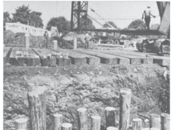
Foundation work is underway for the New York State Pavilion Progress Report #6, September 12, 1962
