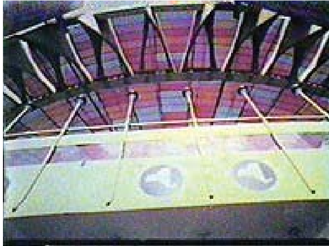
Interior roof appearance.
